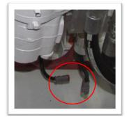
STEP 7) With the hose reel dispensing valve open, plug in the pressure switch to the pump for the hose reel you are purging.
